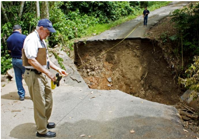
Franklin Lopez from Public Assistance participates in a preliminary damage assessment in the municipality of Barranquitas, Puerto Rico. The severe storms and flooding swept away roads and bridges.
