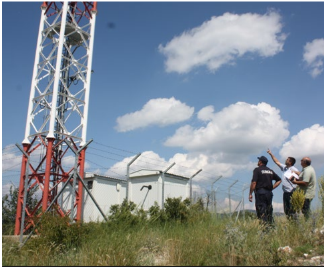
Engineers and representatives from the Ministry of Internal Affairs check the possibility of installing microwave dishes for data transmission on a mast in the village of Polchishte in the municipality of Prilep, 18 July 2018. (OSCE/Gabor Kemeny)
