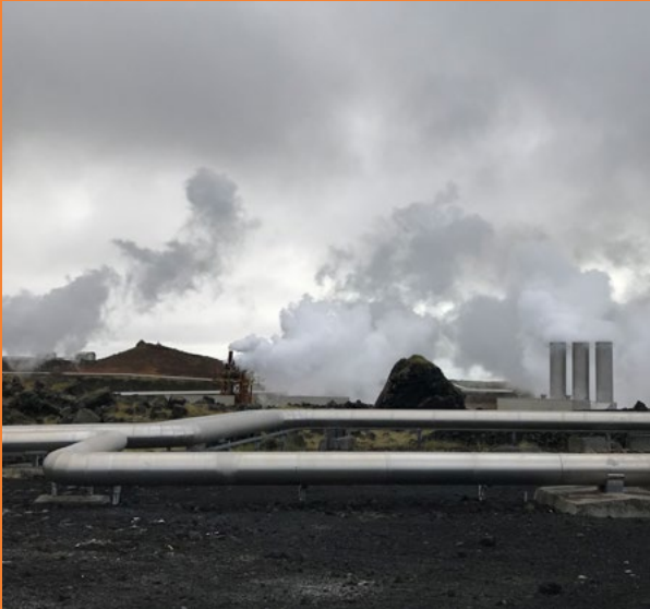
A geothermal power plant in Iceland visited during an OSCE-supported study tour for energy decision makers from several participating States. (OSCE/Daniel Kroos)
